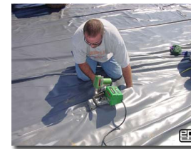
Welding of geomembranes (GM) http://www.geomembrane.com/thermal_welding/index.html
